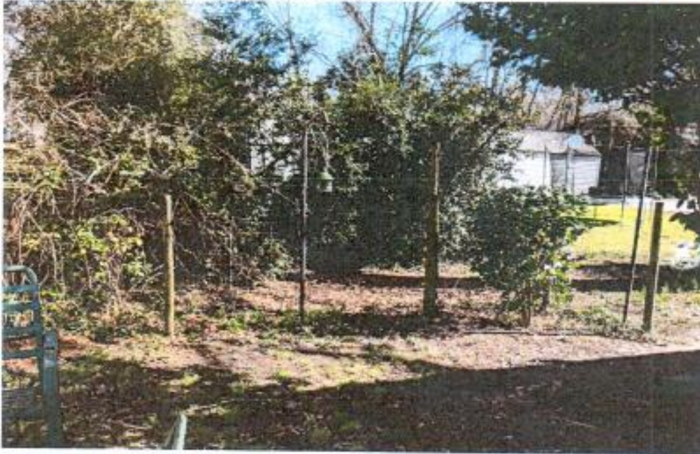
Existing Fence Behind Home- 4 & 5 foot wood posts & hog wire
